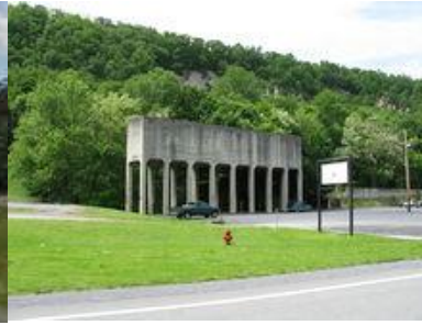
Sand storage bin near sand mines
